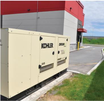
One of the solutions for Benny & Co. includes the KOHLER 100REZGD, 347/600V, 60 Hz gas-powered generator. It also features the KOHLER KSS-ANTA-0200S open transition, automatic transfer switch with weather-protective, sound-attenuated enclosure. The automotive-grade finish helps resist the elements. Kohler Power Systems has delivered energy solutions for markets worldwide since 1920. For more information, visit [KohlerPower.com](http://KohlerPower.com).
