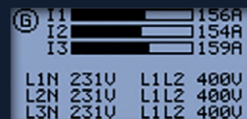
Current and voltage
